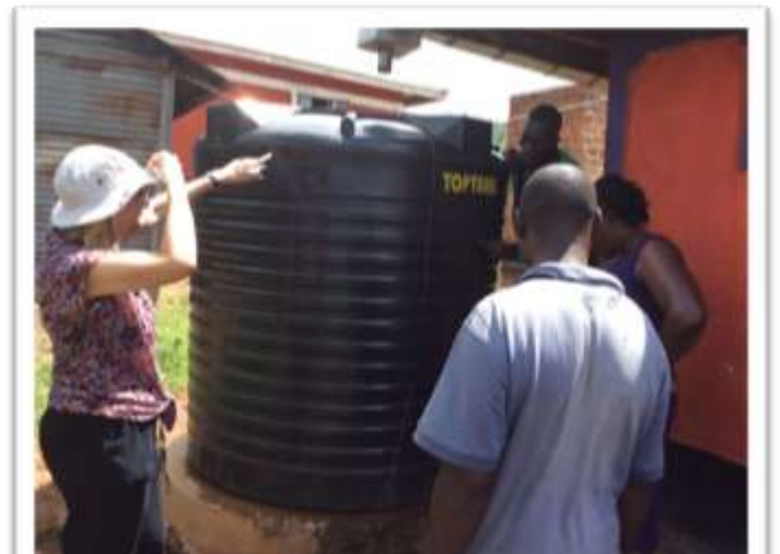
Maintenance checks to the water harvesting system. A precious commodity which is not to be wasted.
